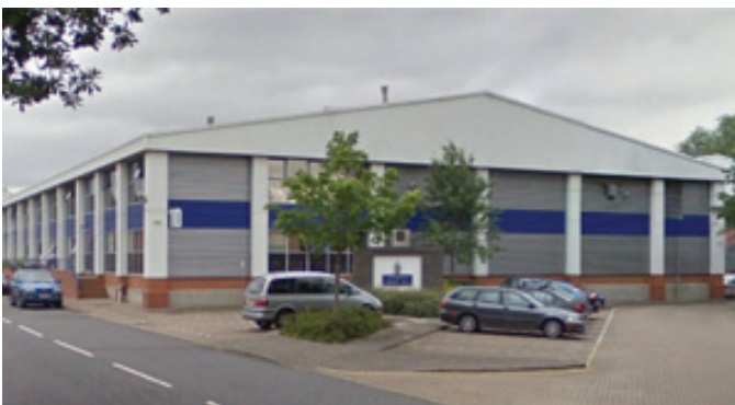
Cam Lock Ltd head office building
